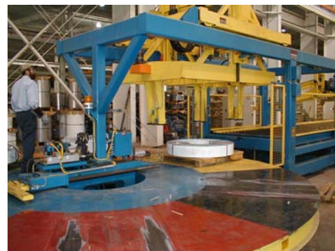
Overhead carriage with VFD
